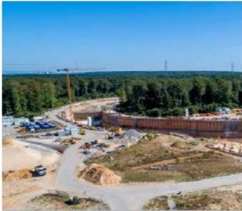
Excavation SIS100 tunnel
