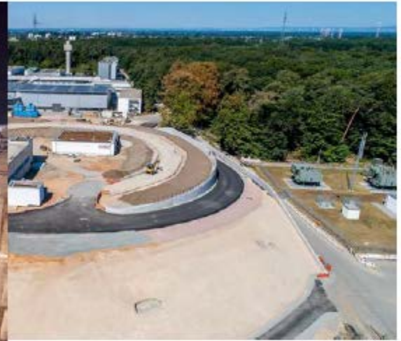
Excavation site prepared ready for FAIR and FAIR phase 0
