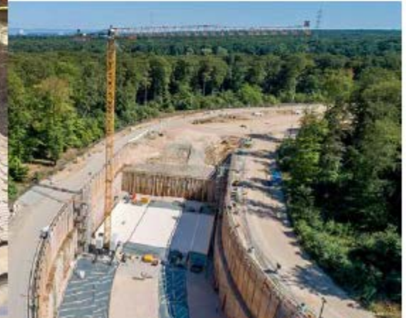
Start of concrete shell works for SIS100
