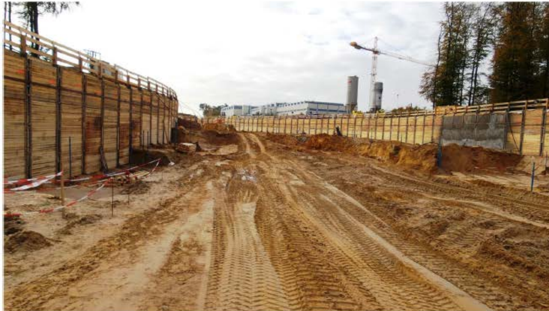
SIS 100: trench sheeting (first 8 meters sheet piling)
