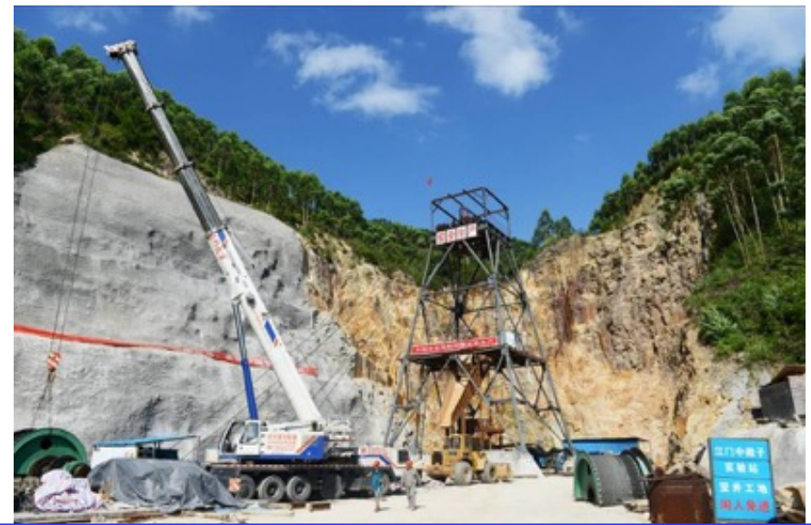
~ 600m vertical shaft, ~1300m sloped tunnel All blasting completed on Dec. 30, 2020, water pool construction on the way
