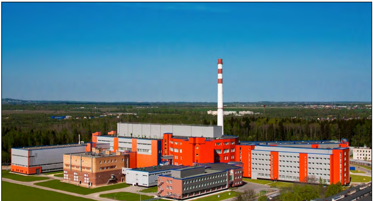
Fig. 1. Overall view of the PIK reactor complex
