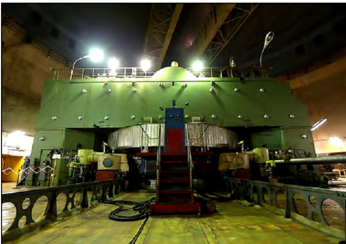
Fig. 1. General view of the 1 GeV proton synchrocyclotron (SC-1000)
