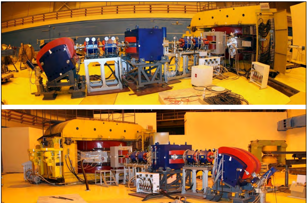
Fig. 1. General view of the C-80 cyclotron
