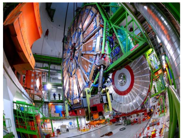
Fig. 12. The lowering down of one iron disc with muon chambers in the underground hall
