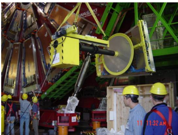
Fig. 11. Installation of a muon chamber on the iron disc of the magnet return yoke
